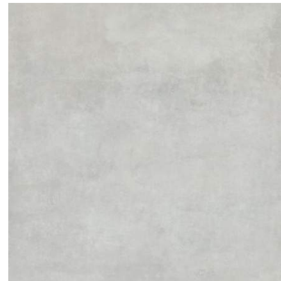
CHIMNEY - PARGED CONCRETE
