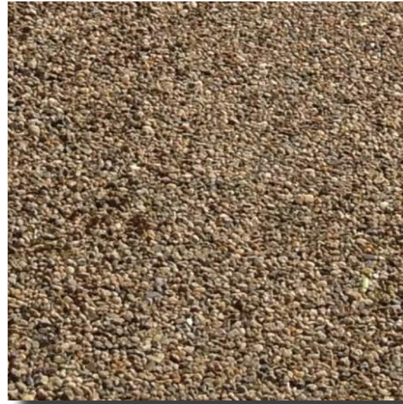
IMPERVIOUS WALKWAYS - TAN CHIPSEAL
